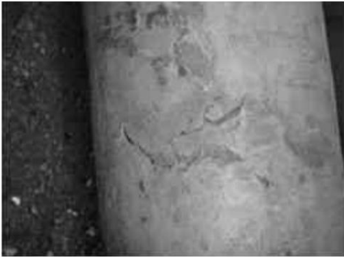
Figure 1 - Surface cracks of forging
